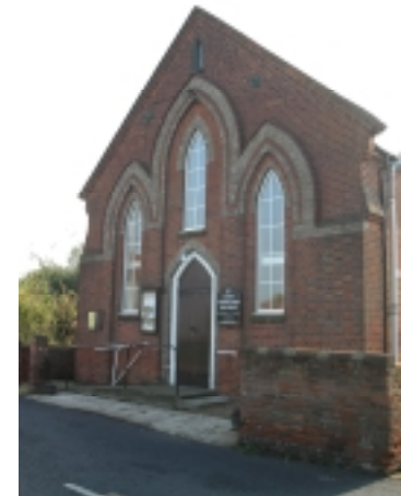
STUTTON METHODIST CHURCH Manningtree Road Stutton Suffolk
